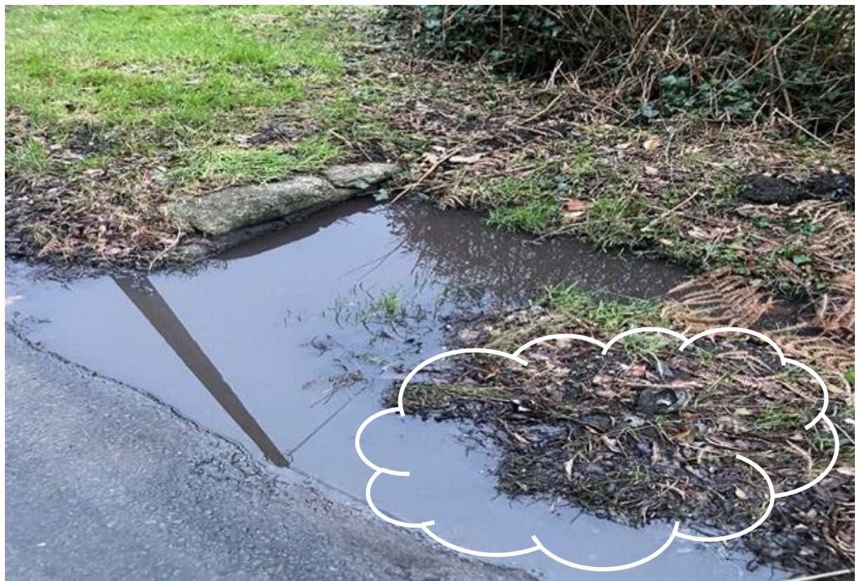
Blocked culvert, oily water, and underlying soil staining.
