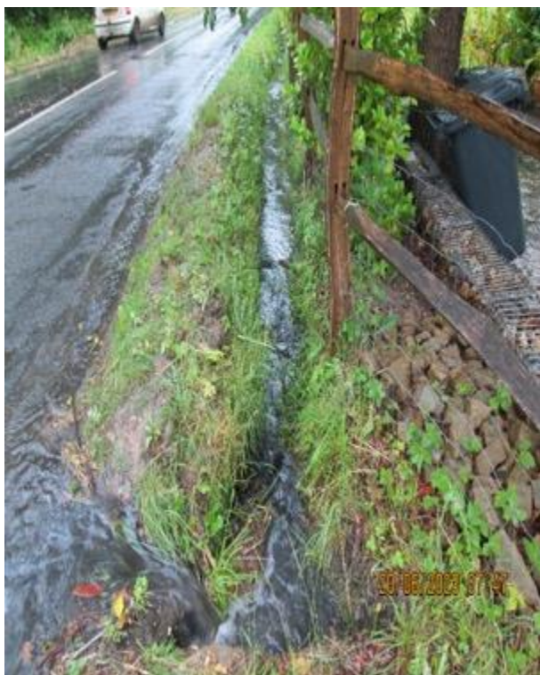
Oil-laden water bypasses the culvert.
