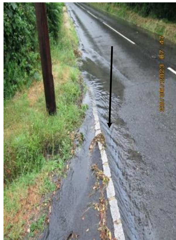
Water from ditch by-passing culvert (Oil noted).
